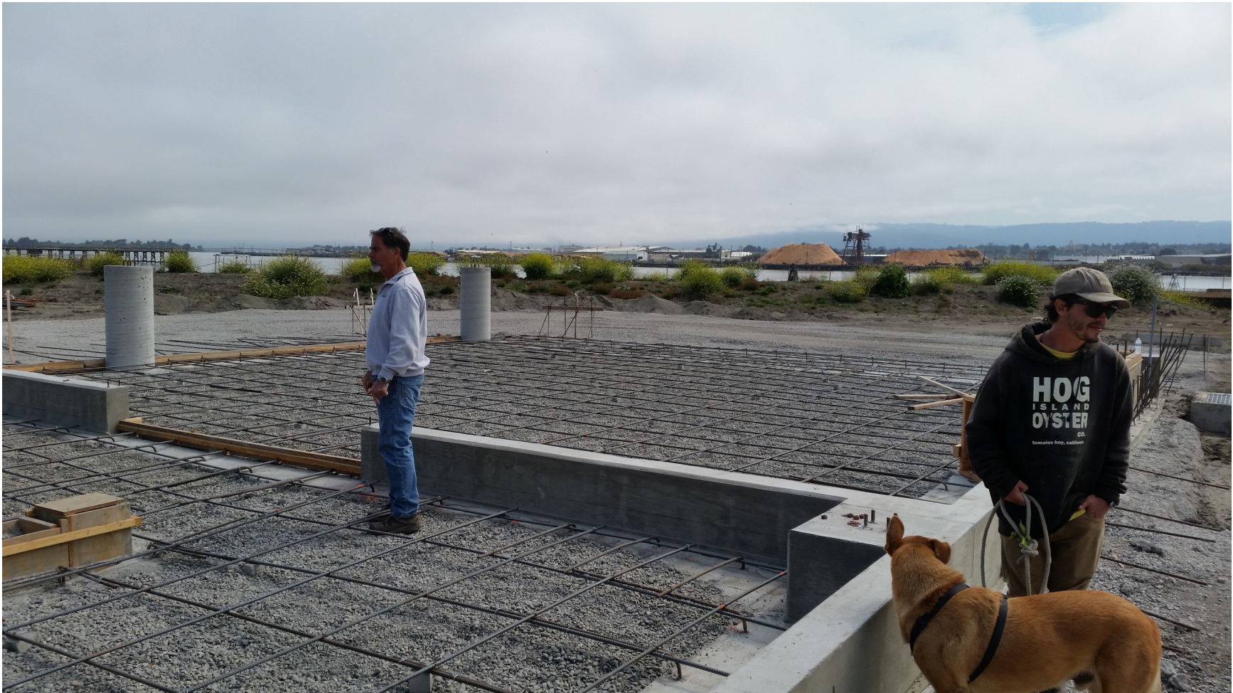
Figure 6. Construction site of Hog Island Oyster Company hatchery on Humboldt Bay, with Terry Sawyer (left) showing the approximate location of the Burkolator and lab bench within the building.
